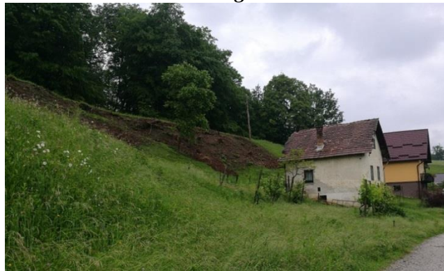
Figure 2: The landslide endangered the houses in the near.
