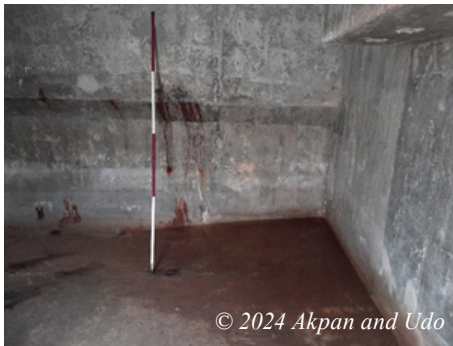
^ Image 22: Water seeped within the Bunker
