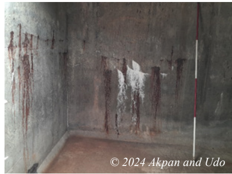
^ Image 23: Rusted Inner walls of the Bunker
