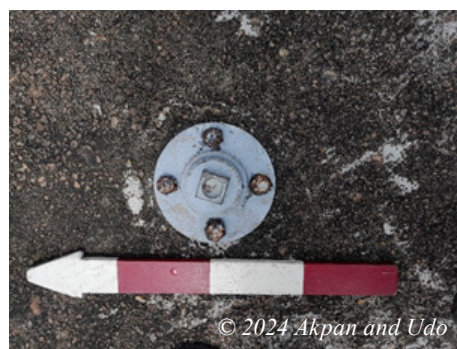
< Image 28: Close view of the closed Air Vent
